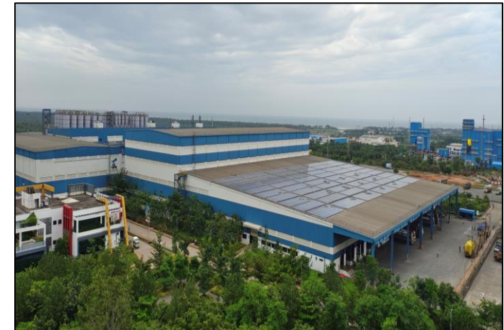
1MWp Solar rooftop power plant
